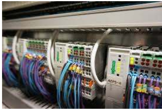
Programmable Logic Controllers mounted on a cable tray connected via Ethernet
